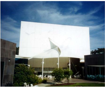
The wall attachment is a series of short SS Cables connecting to a catenary edge to both membranes. The overlap was designed to add an element of weather proofing and play of light and shade.
